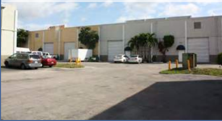
Kelsey Business Center at Park Road
